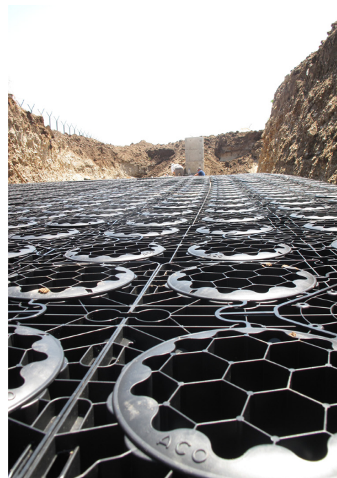
Final result: 4 installers x 6 working hours = 75 m 3 ACO Stormbrixx
