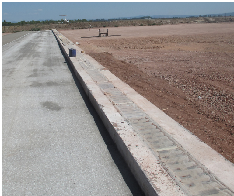
Heavy-duty channels ACO Monoblock during the installation
